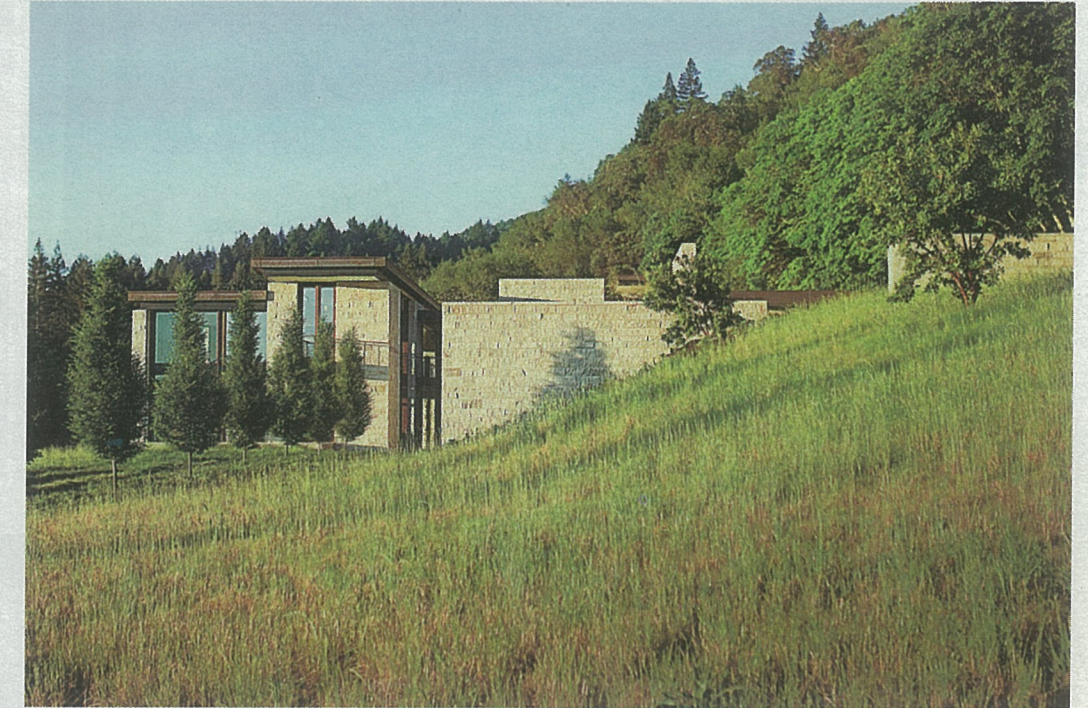
Above: Aidlin Darling Design's large split-face sandstone-clad Wine Country house is divided into public (vineyard-facing) and private wings tucked deftly into the hillside; left, from poolside in back, the glassy dining room seems like a bridge between the wings divided by a reflecting pool that runs north to south.
