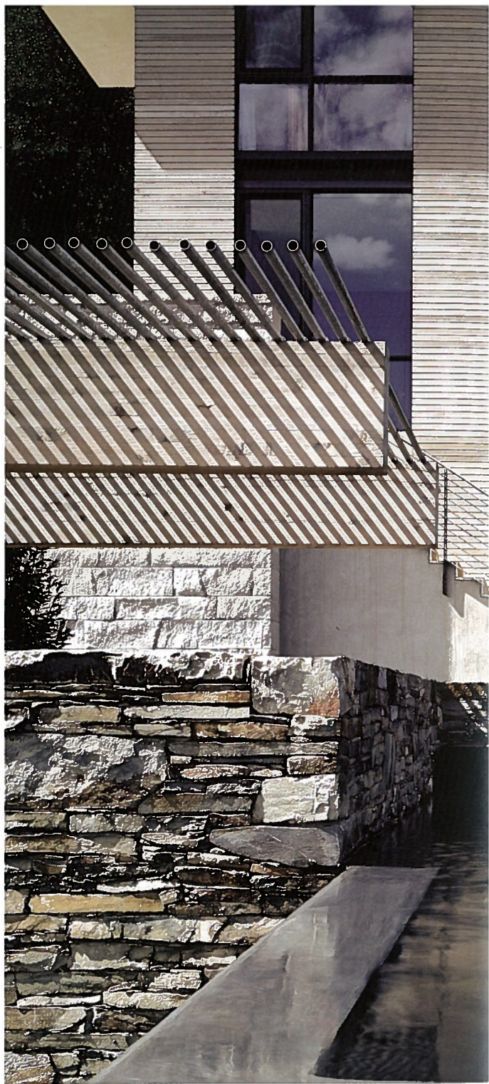
就餐區上方金屬與木頭搭建的花架可以緩和夏天強烈的陽光。同樣充滿了圖形設計感 Metal and wood trellis over dining terrace modulates the intensity of the strong summer sun and provides graphic shadow patterns. (Photographer: John Sutton / Jamie White)
